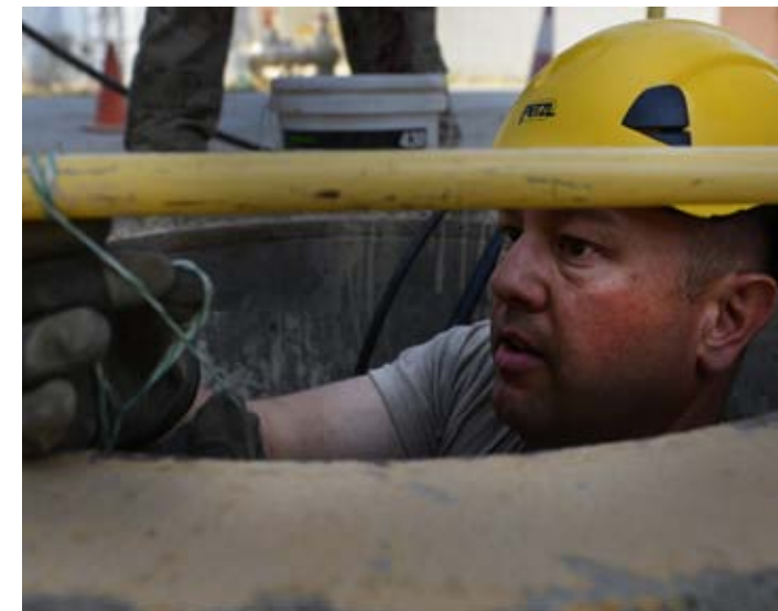
Staff Sgt. Lawrence Santos installs a cable shoe May 15, 2014, at Bagram Airfield, Afghanistan. The cable shoe will help prevent damage to the cable from rough or sharp surfaces. Santos, a East Taunton, Mass. native is a Combined Air and Space Operations Center Engineering and Installations cable and antenna technician, deployed from the 212th Engineering and Installation Squadron, Otis Air National Guard Base, Mass. (U.S. Air Force photo/Senior Airman Sandra Welch)
