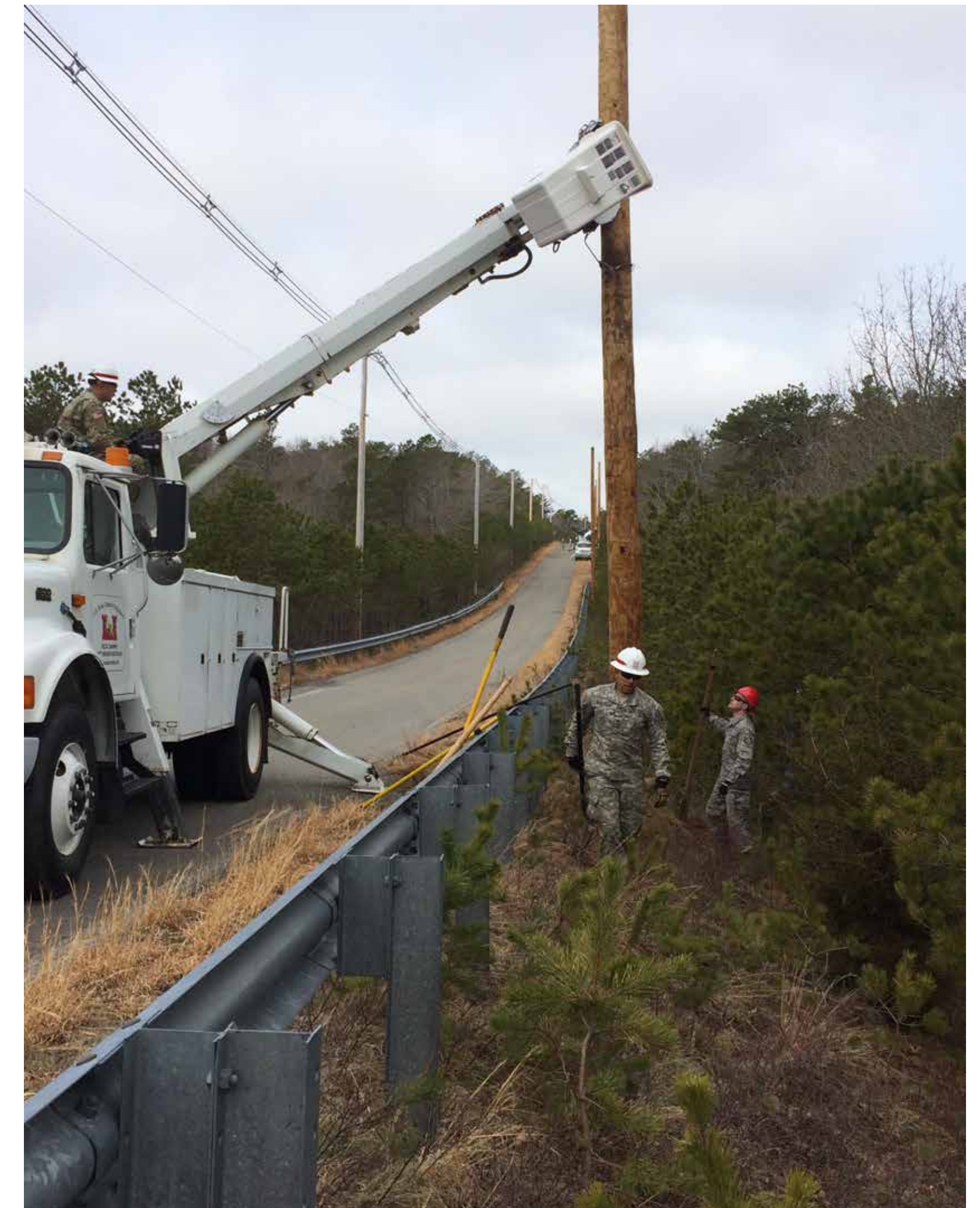
(left) Military leaders and civilian consultants confer on details of the work in progress and talk about the next phase plans based on what was learned in the shakedown weekend. (right) ANG and Army line crews cooperate to set 22 new 45-foot utility poles in Phase 1 of the 3.5 mile overhead line construction taking place over 2 years. (photos courtesy of Maj. Shawn Doyle)
