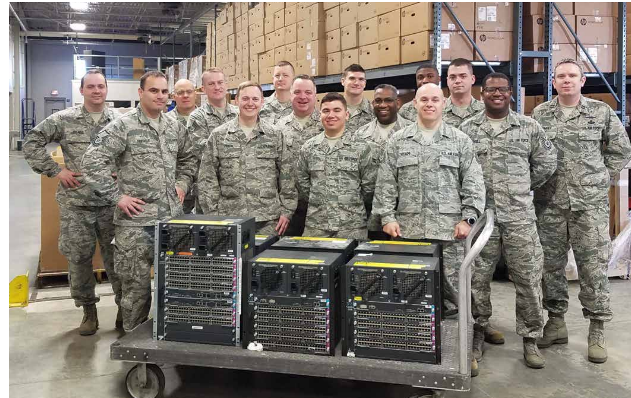
15 Air National Guard Cyberspace Engineering and Installation Airmen descended on Joint Base McGuire-Dix-Lakehurst in New Jersey for two weeks to upgrade the base's network. The team was assembled from Airmen representing 9 individual units from multiple states across the country.
