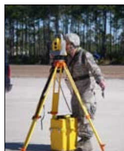
Staff Sgt. Peter Kurt, 102nd Civil Engineer Squadron, sets Precision Approach Path Indicator Lights (PAPI) during Silver Flag. The tolerances are restricted to within 1-inch elevation and distances from the threshold are essential, requiring very accurate calculations.
